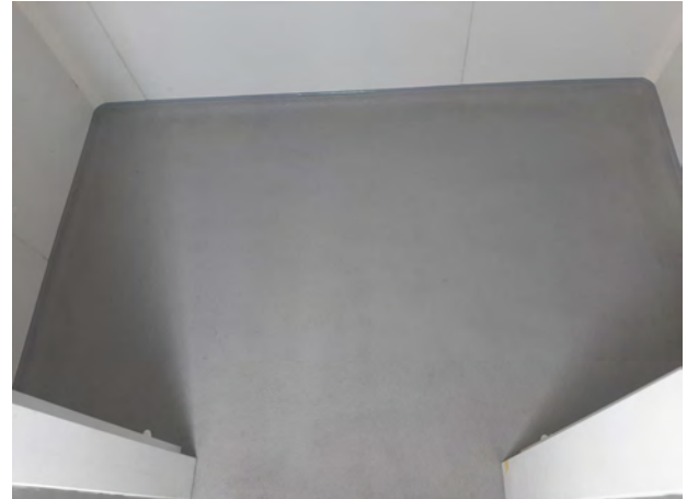
Hygienic Solutions MMA Colour Quartz System with Specially Designed Coving System for Cold Room & Freezer Rooms
