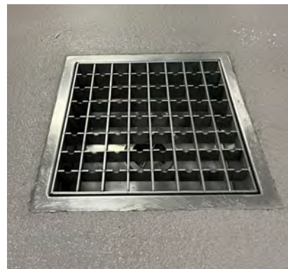
Hygienic Solutions Stainless Steel Drain Applied within a kitchen.
